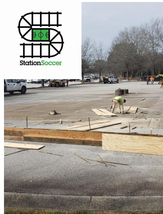
Station Soccer Broke Ground in February at Kensington Station
